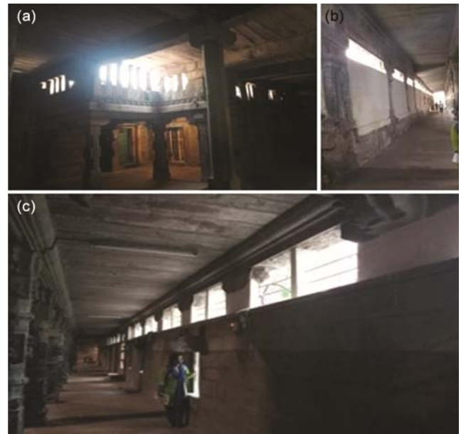
Fig. 3 — The figure (a) showcases the provision of clerestory window in Nellaiappar shrine, figure (b) displays the clerestory windows near "kaatchi mandapam" figure (c) Clerestory Window in Chain mandapam (sangili mandapam)
