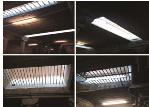
Fig. 6 — Images of different chimneys portraying the ventilation mechanism in Nellaiyappar shrine (Source: Author)
