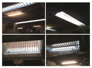
Fig. 6 — Images of different chimneys portraying the ventilation mechanism in Nellaiyappar shrine (Source: Author)
