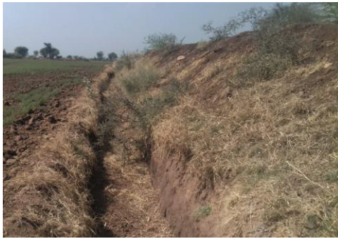
Fig. 8 — Trench with soil bund
